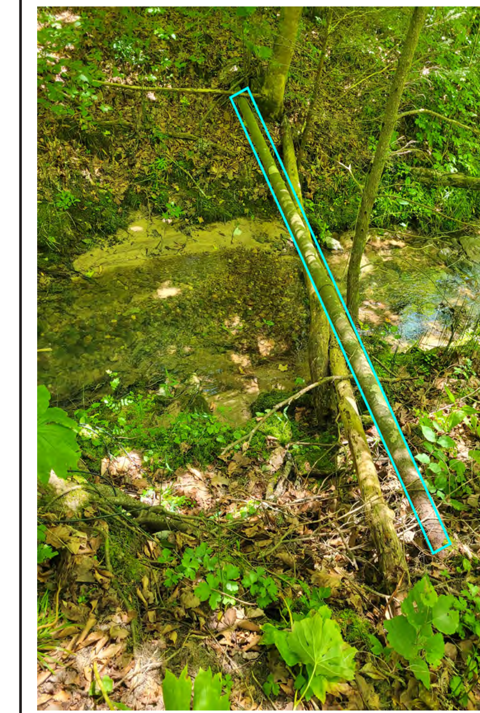
Figure 5. Pipe a few feet downstream of Site 8.
